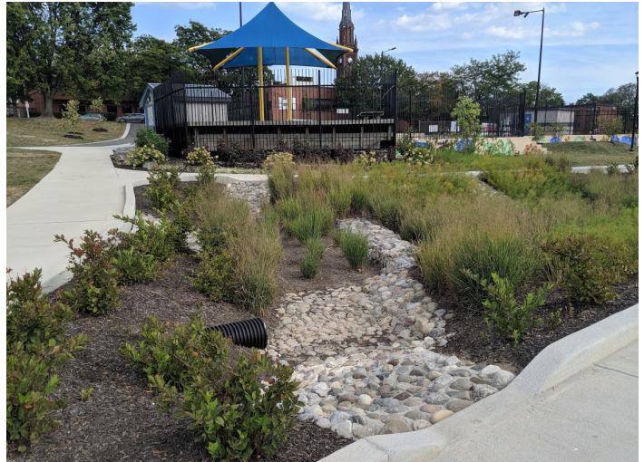
Henrietta Lacks Educational Park in Baltimore, Maryland, showcases green infrastructure elements such as this bioretention feature. Photo courtesy of NRPA
